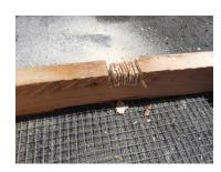
2. Using an electric skill saw set at a depth of 2.5 cm, make many cuts within the 5cm section.
